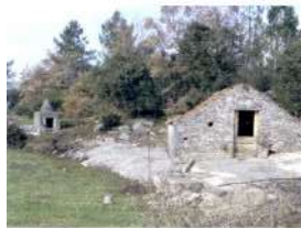
Cisterns (water tanks)
