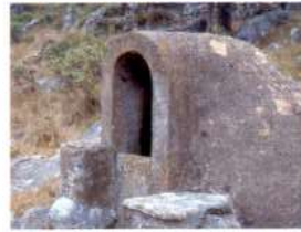
Cistern (water tank)
